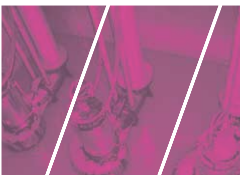
Wastewater Transport and Treatment
