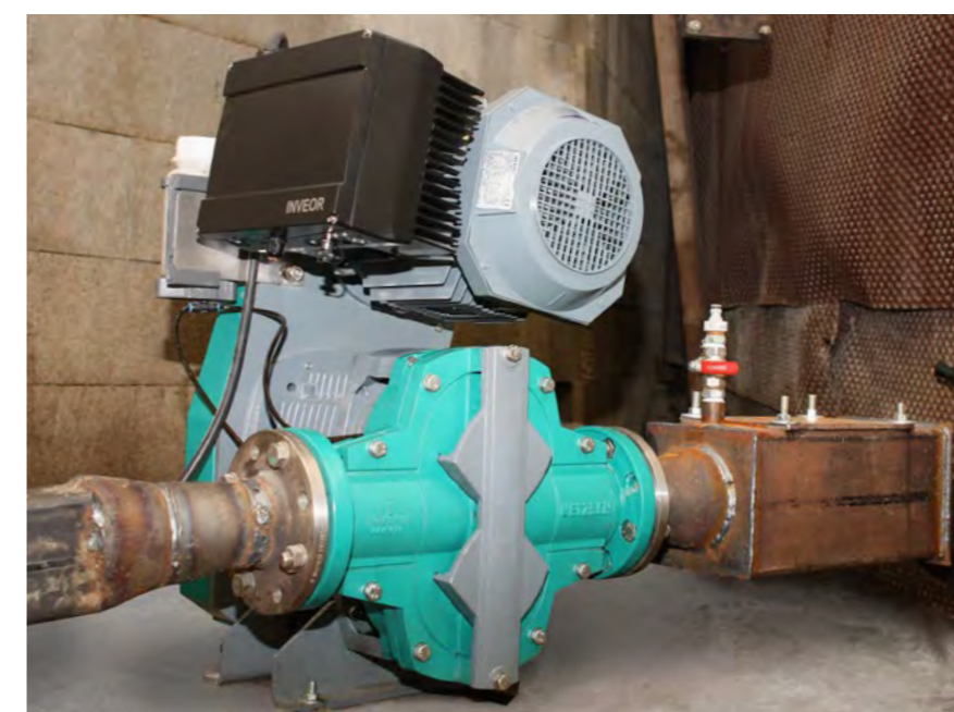
Recirculating liquid manure in a biogas plant from a fermenter to a heat exchanger at a flow rate of 20 m 3 /h against a discharge pressure of 1,5 bar.
